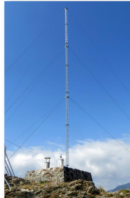
Modernised transmitting antenna IALA Beacon BEAR
